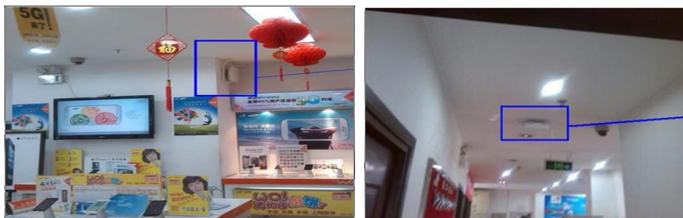
Figure 4-1 pRRU installation position
