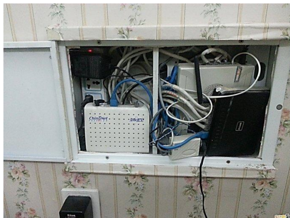
Figure 3-2 Information boxes housing home gateways have metal plates
